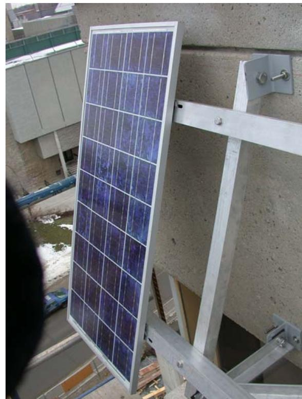
Fig. 11. Aluminum support structure used to attach the PV awnings to the building.
