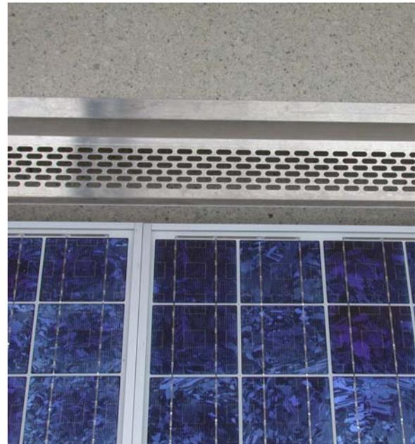
Fig. 13. Photo of the baffle/flashing used above the PV arrays.
