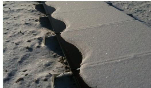
Figure 8 Non-uniform shading pattern created by snow
