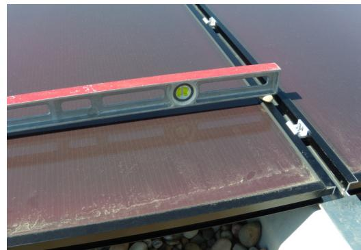
Figure 2 Soiling pattern reveals a side-to-side tilt and hints at the true azimuth.
