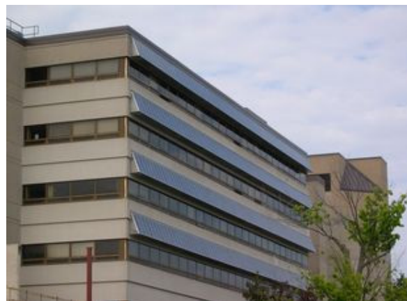
Fig. 1 Goodwin Hall photovoltaic array
