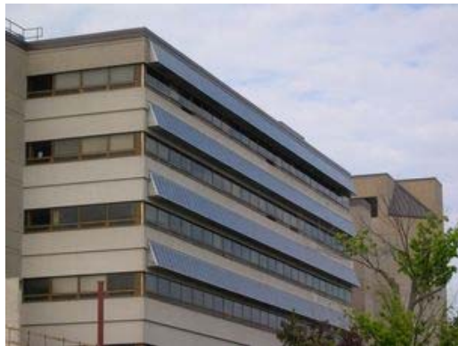
Fig. 1. Goodwin Hall photovoltaic array
