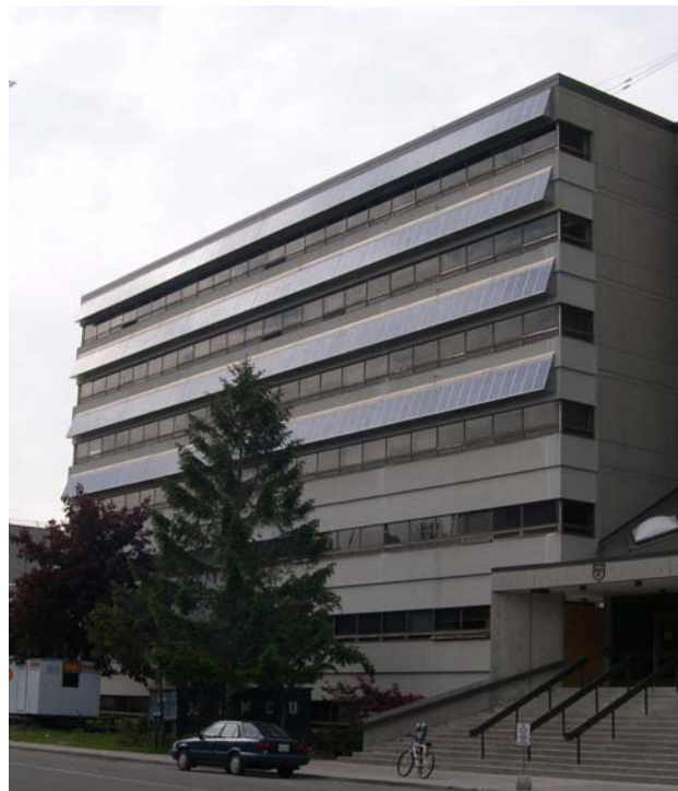
Fig. 1. The building integrated photovoltaic (BIPV) system installed at Queen's University.
