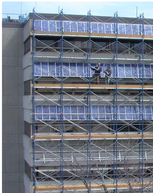
Fig. 12. Installation of the PV arrays on the building.
