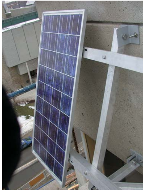
Fig. 11. Photo of the aluminum support structure used to attach the PV awnings to the building.
