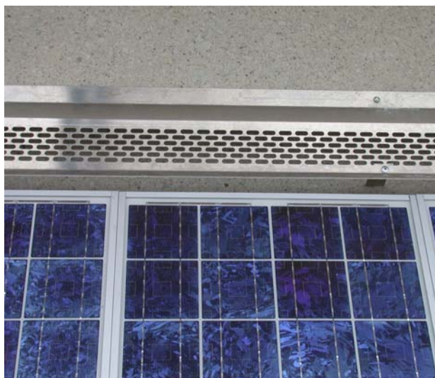
Fig. 14. Photo of the baffle/flashing used above the PV arrays.
